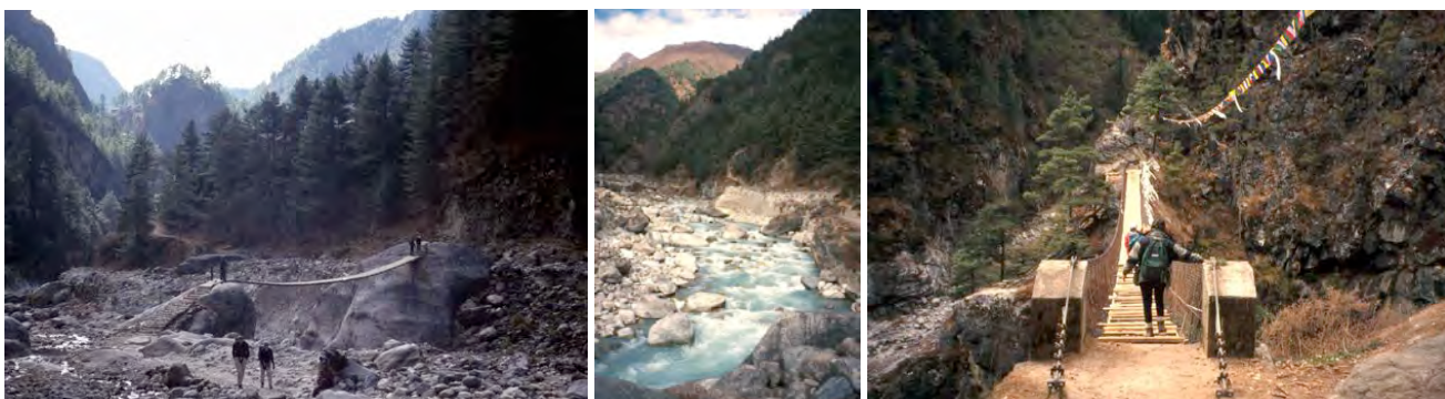
Left to Right: a low suspension bridge (near lunch spot), approaching climb to Namche, the highest suspension bridge
